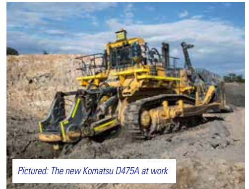
Pictured: The new Komatsu D475A at one of the work sites.
