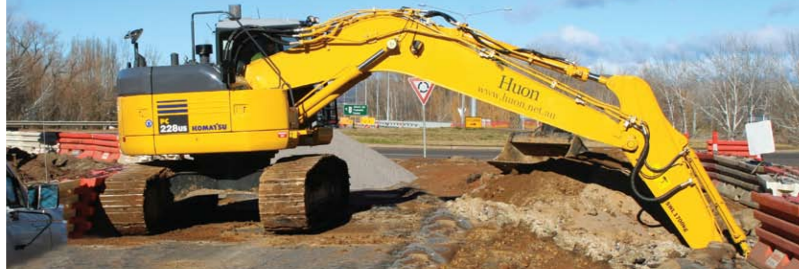
ABOVE. Komatsu's PC228US-3 excavator carries out road upgrading maintenance work.
