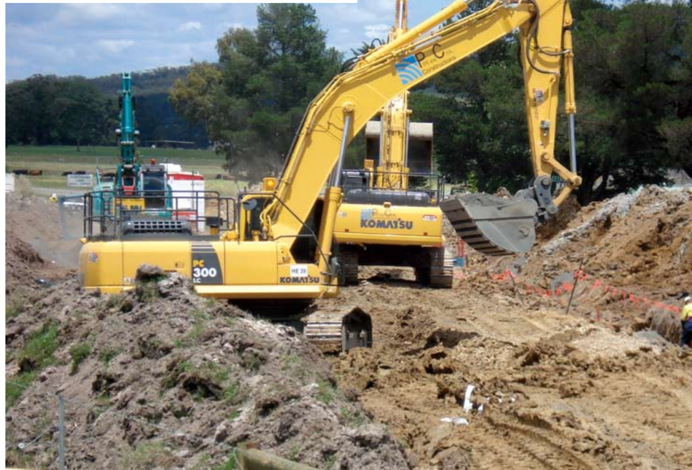
ABOVE/RIGHT. Victoria's Sugarloaf Pipeline Project.
