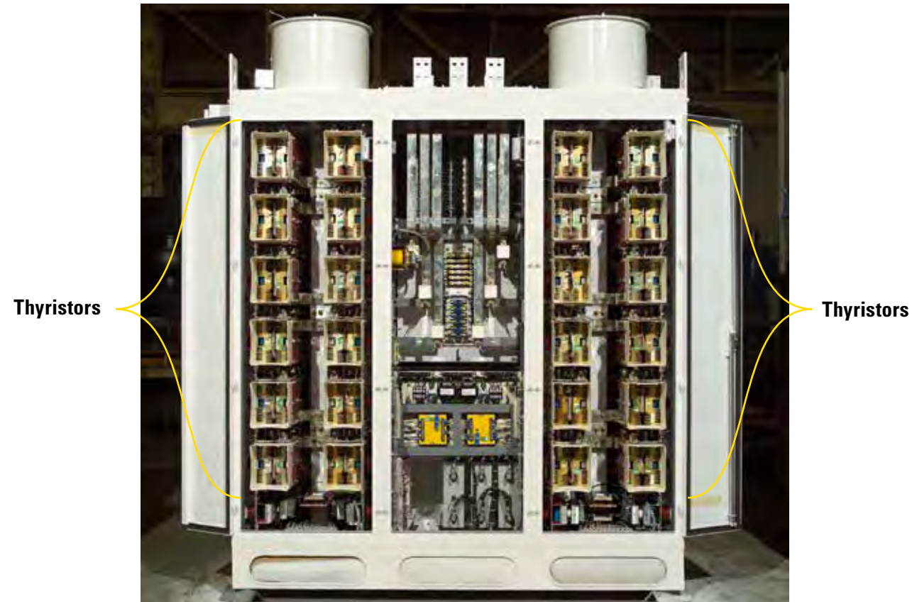
Figure 44 The converter cabinet houses the thyristors used in converting AC power to DC power. The P&H Electrotorque system returns 10% to 15% of the original electrical energy through regeneration to the mine distribution network in the same pattern as the three-phase AC supply.
