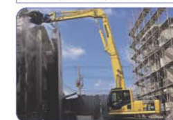
Super-long boom and arm for demolition
