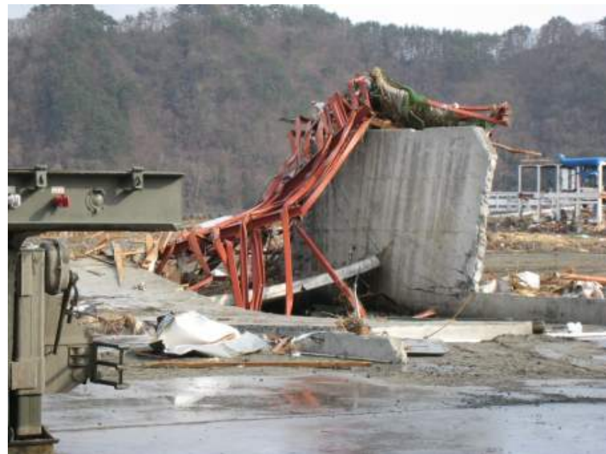
Kamaishi Branch of Komatsu Iwate Ltd.
