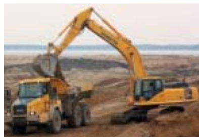
PC300LC hydraulic excavator and HM300 articulated dump truck in operation
