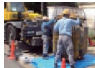
Transformers being removed from the Osaka Plant for disposal
