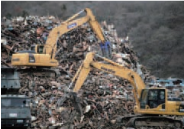
Hydraulic excavators at work in stricken area
