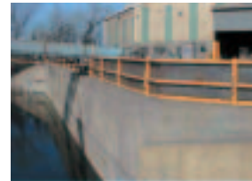
Fence to prevent rainwater from flowing into the creek
