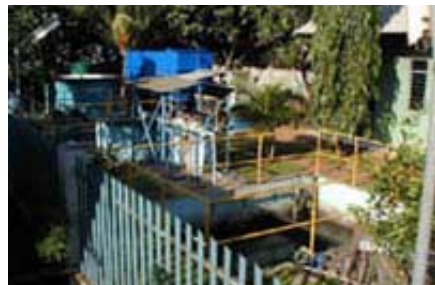
Final water treatment plant
