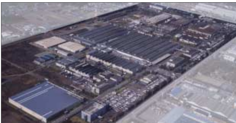
⑤ Oyama Plant, the model manufacturing facility for zero emissions activities.
